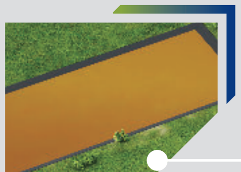
Leachate Collection Pond
